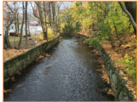
2007 overbank floodwater height ~ 6.3 ft above 1936 laid stone wall
